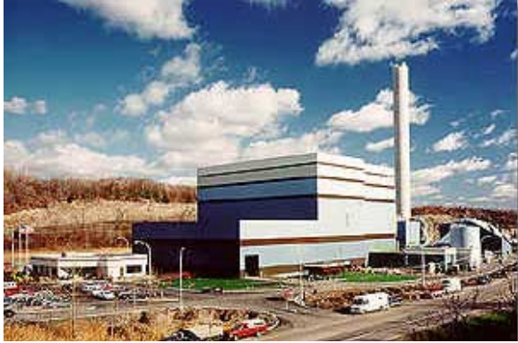
Figure a - Onandaga County Waste to Energy Plant
